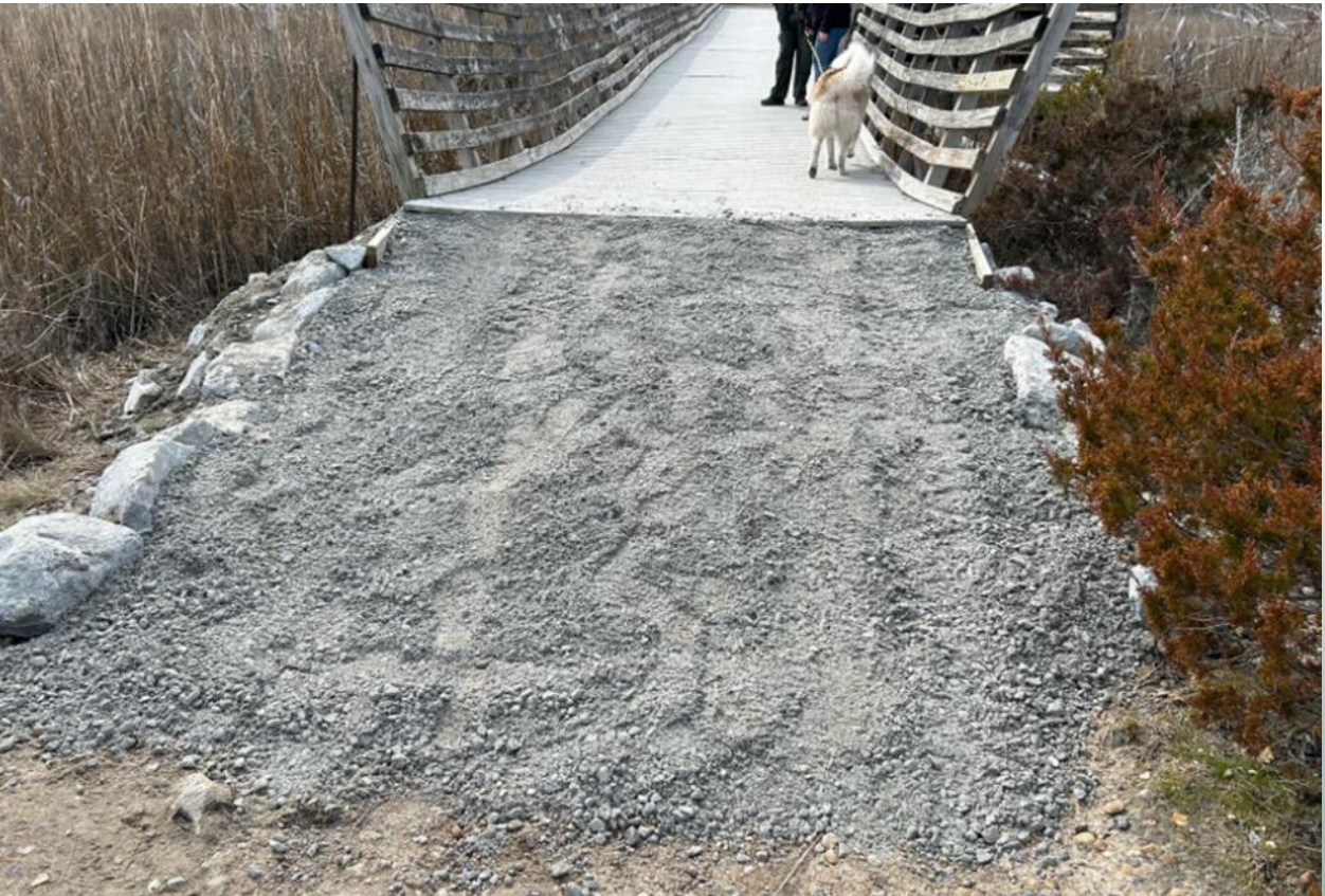
Marsh Bridge approach (after Day 1, Feb 16)
