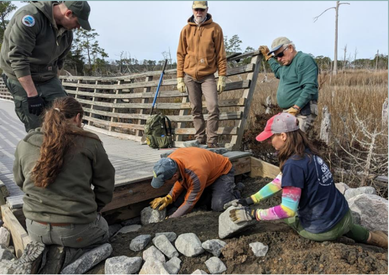
The team dug out old material and placed rip rap to build up a new ramp
