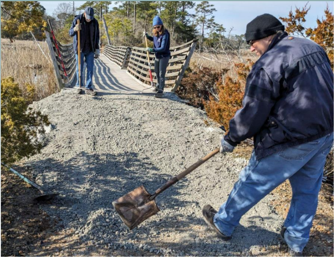
Marsh Bridge approach (after Day 2, Feb 22)
