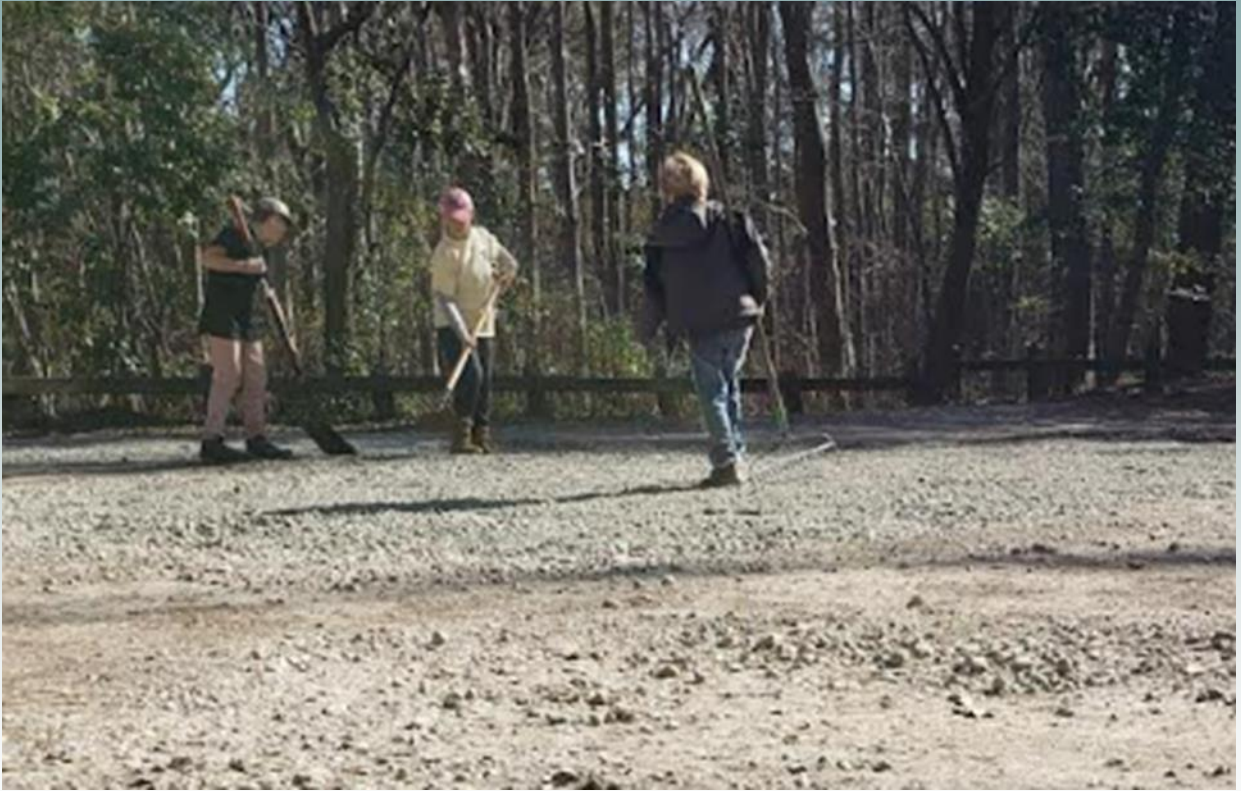
Spreading and leveling out the crusher run.
